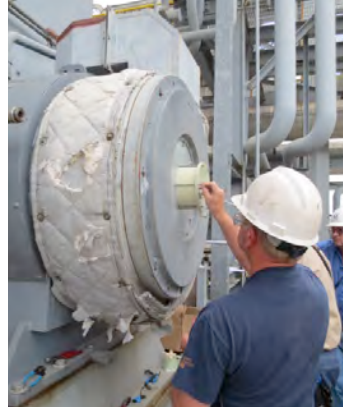
Figure 3 – Installations of EFREM on GE 7A6 units
